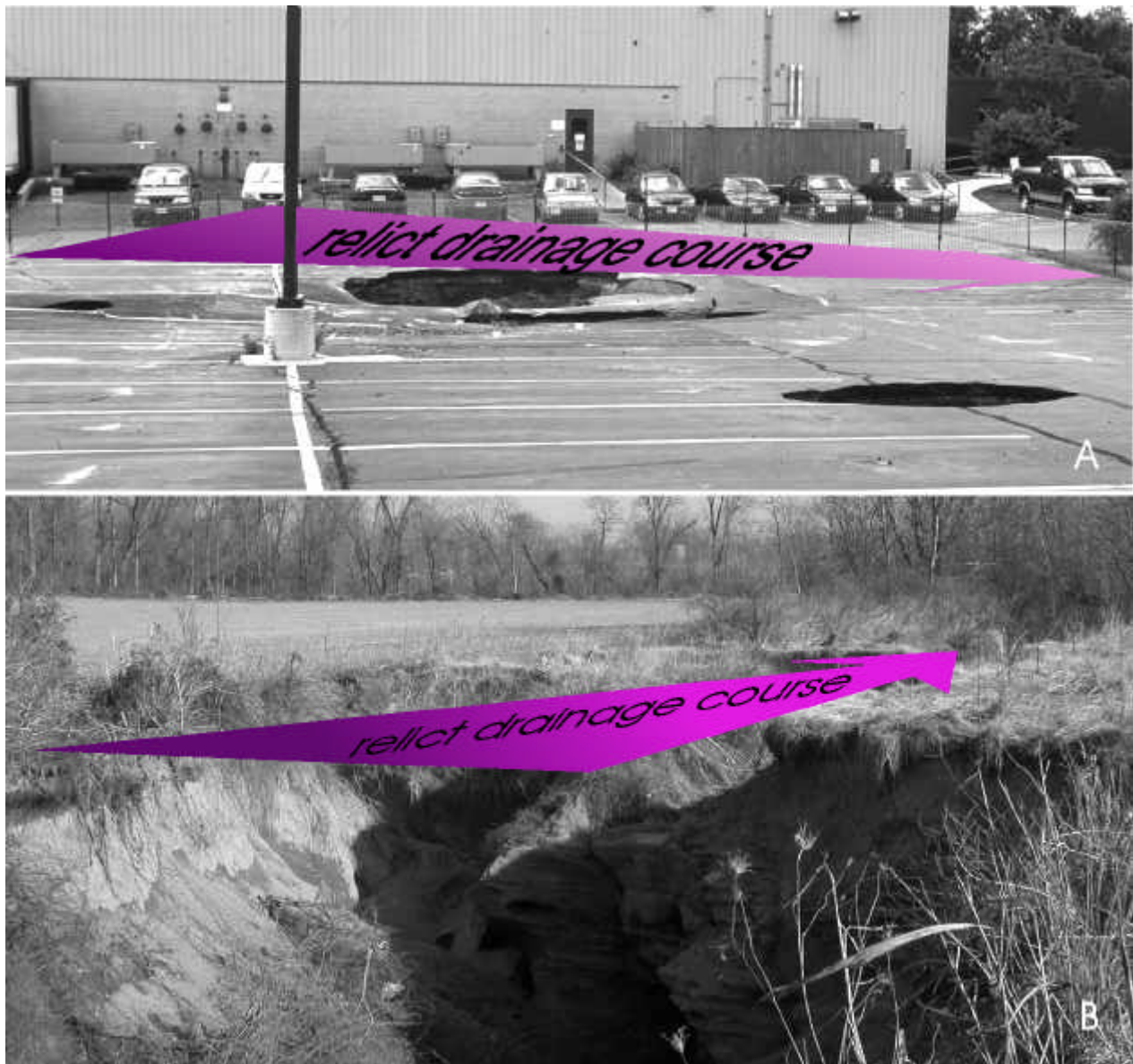
Figure 33. – Some examples of drainage lowlands acting as sites of sinkhole activity. A, Parking lot present in the Ceresville Member of the Grove Formation in northeast City of Frederick collapsed along prehistoric drainage area. B, Coalescing sinkholes in the Lime Kiln Member of the Frederick Formation created along drainage lowland in southeast City of Frederick.
