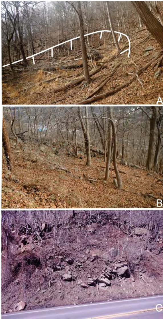
Figure 25. Segments of rotational slumps at Luke, Maryland. A, Arcuate scarp of a single rotational slump. See Figure 24A for location. Note disturbed vegetation from unstable slope. B, View of the nearly flat upper surface of an individual slump. C, Toe of an individual slump as seen along MD Route 135.
