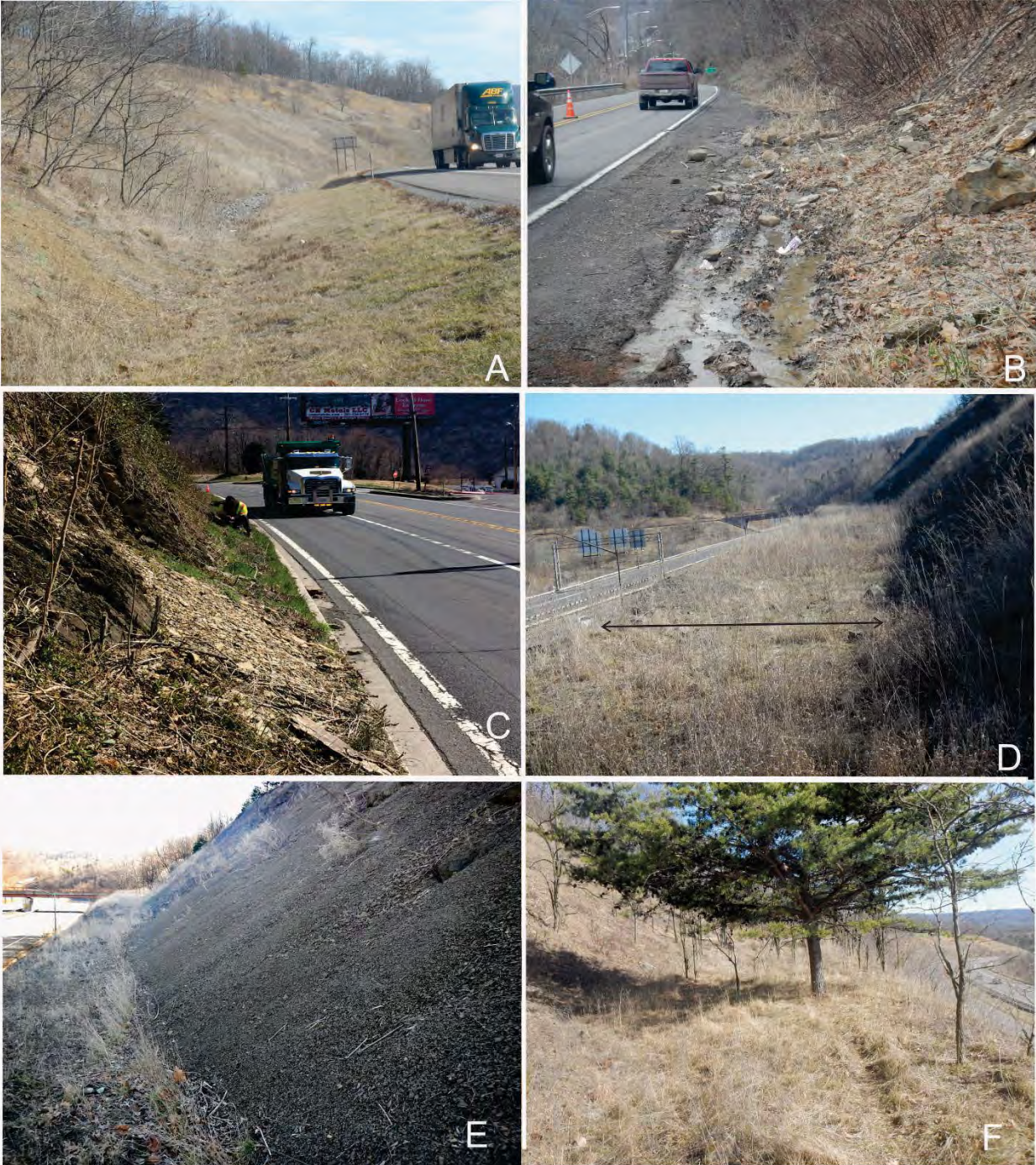
Figure 9. Benches and catchments styles and character. A, Catchment shoulder sloping away from the roadway. B, Flat catchment shoulder. C, Shoulder inclined towards the roadway. D, Elevated catchment bench clear of debris. E, Elevated bench nearly filled with debris. F, Elevated bench with woody vegetation.
