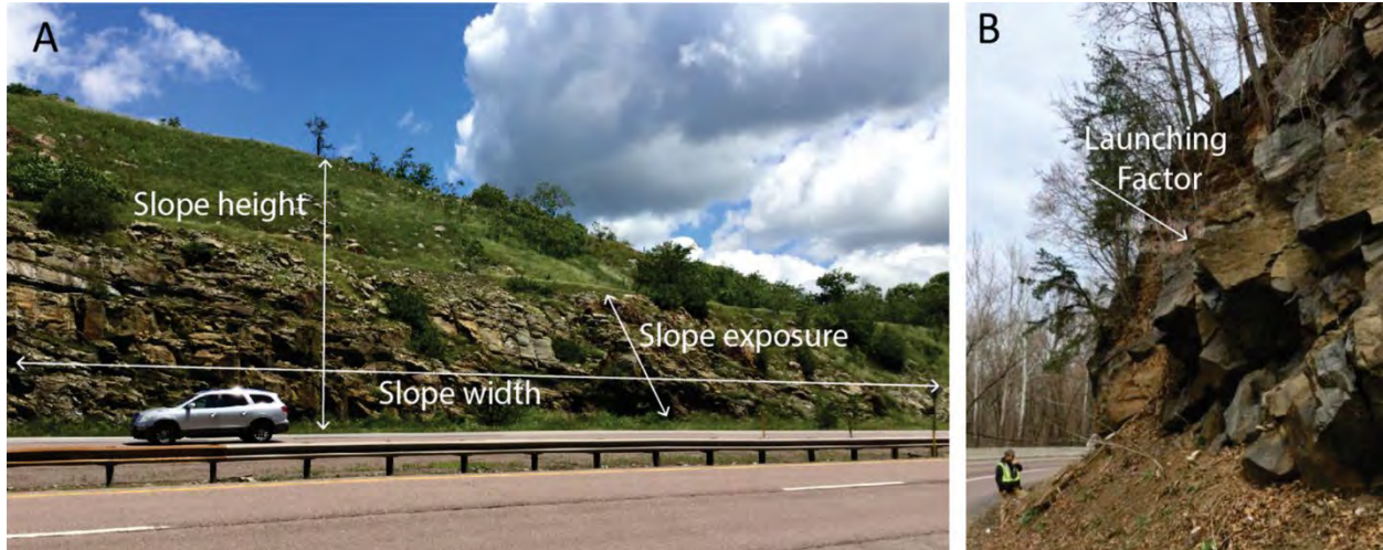
Figure 8. Embankment characterization. A, Slope dimensions. B, Launching factors.
