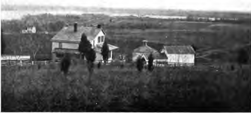
FIG. 1.—VIEW SHOWING SUNDERLAND TERRACE WITH LAFAYETTE FORMATION IN THE FOREGROUND, ELKTON, CECIL COUNTY.
